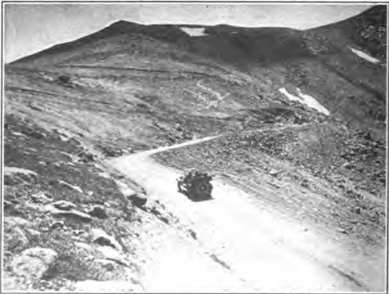
The Finished Road.
